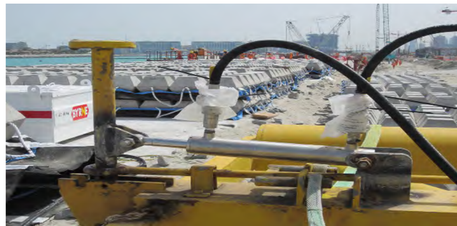
Deepwater Frame deploying Uni-Flex mattress with anchoring attachments
