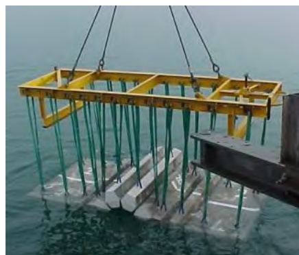
Deepwater Frame deploying Uni-Flex mattress with anchoring attachments
