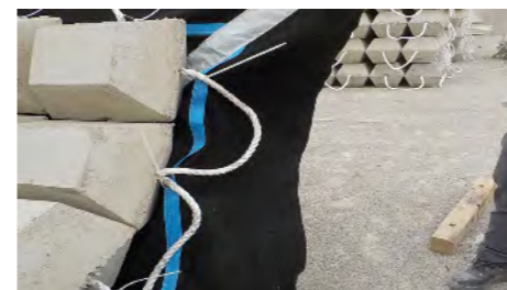
Overlay flaps for total geotextile cover
