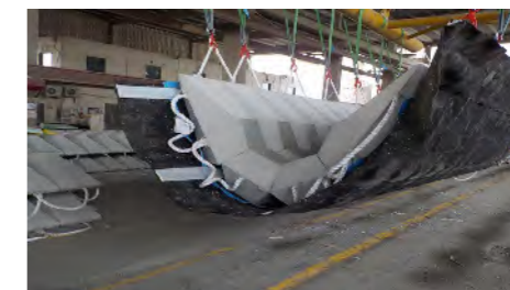
Stiffener rods for diver free installation
