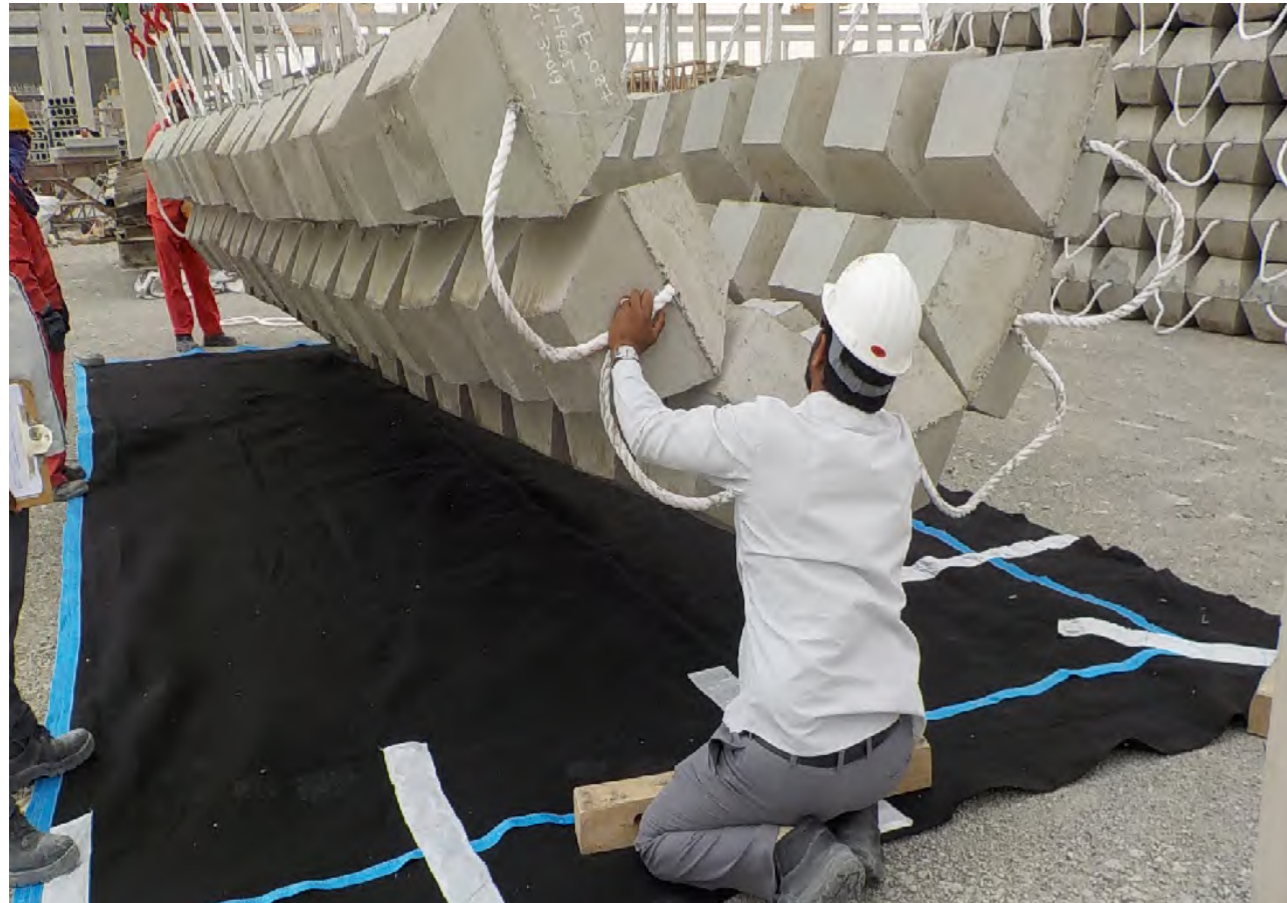
GEO=MAT can be pre-fixed to either side of the concrete mattress or even both sides.
